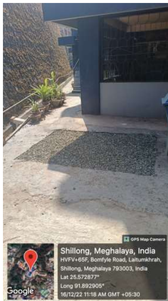
Borewell recharge at Shillong College, Main Campus
