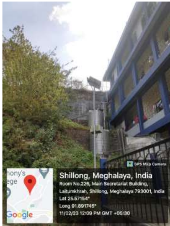
Solar Street lights at the Girl's Hostel, Shillong College
